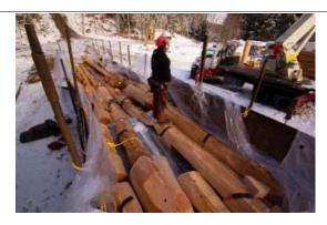
B.C. Each piece used in the construction is carefully numbered — the lakeside home has about 1,500 — before the homes are taken apart and shipped to the build site. "(The numbering) is unbelievably important, especially on the other end when they're setting it up," says crane operator Danielle Haynes. "They have to know where each log goes."
