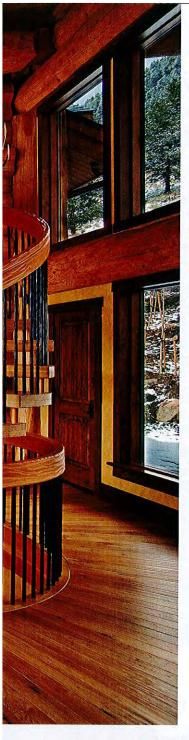
**LEFT:** Gunter crafted the radiating treads for the circular staircase from Douglas fir boards that Pioneer Log Homes sent with the logs, including the 53-foot-tall center post.
