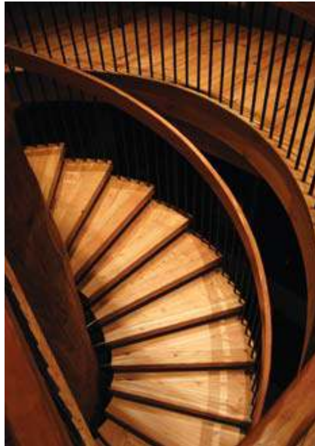
Left and Below: Along with the cedar logs, Pioneer sent Douglas fir timbers and Gunter, using a CNC machine, crafted the planks for a circular staircase to the tower room, which serves as the home office. In addition, there is a suspended bridge above the main foyer that adds even more character to the area.
