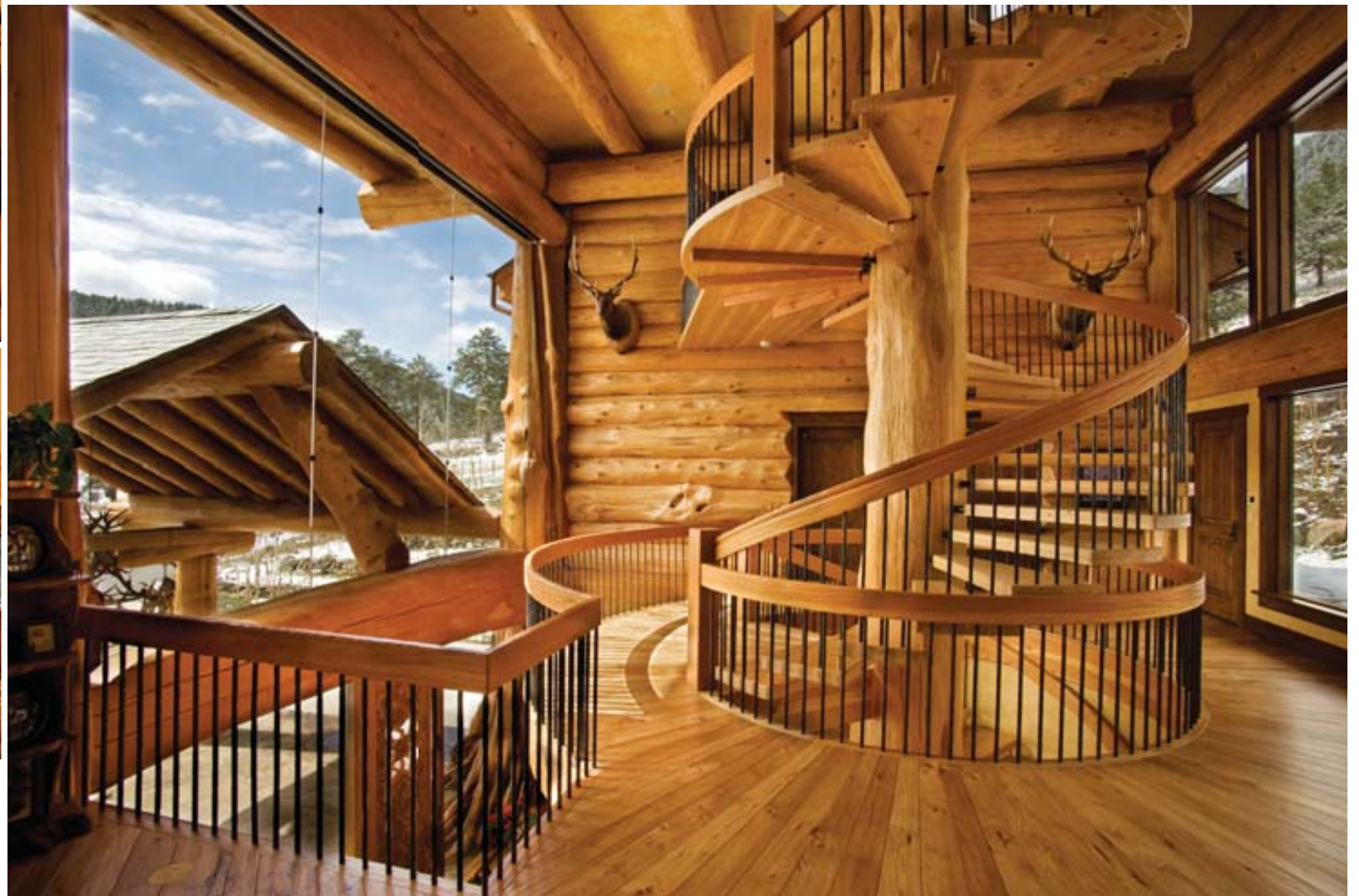
Left and Below: Along with the cedar logs, Pioneer sent Douglas fir timbers and Gunter, using a CNC machine, crafted the planks for a circular staircase to the tower room, which serves as the home office. In addition, there is a suspended bridge above the main foyer that adds even more character to the area.
