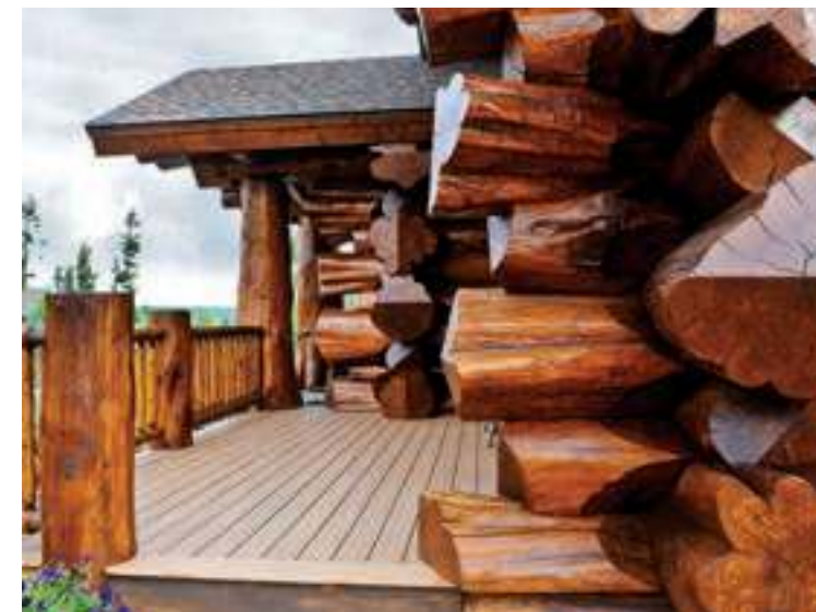
ABOVE: Staggered log ends and scribe-fit corner notches give the home truly handcrafted style.
